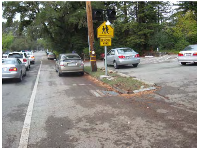
Figure 2. Westbound Woodside Road in front of Church parking Lot
